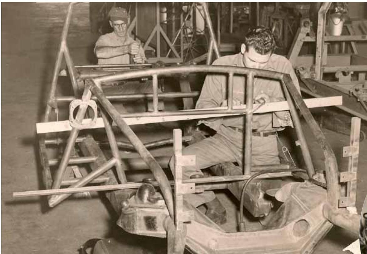
Above: The integrated roll bar on this chassis indicates that it is s/n 5206, the only coupe bodied in West Palm Beach. After the first car, all Cunninghams utilized Chrysler's 331 cu. in. Hemi with a log manifold designed and built by Cunningham.
